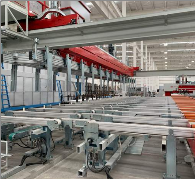
Figure 7. The automated stacking system moves profiles from the table and loads them into baskets for aging.
